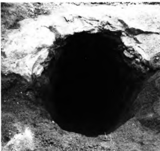
Photo. 5. 45° Shaft for delivery main
