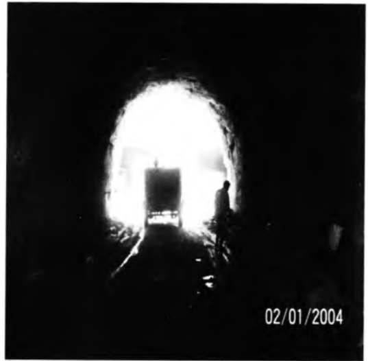
Photo. 8. View from inside the tunnel
