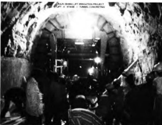
Photo. 11. Lining work in darkness
