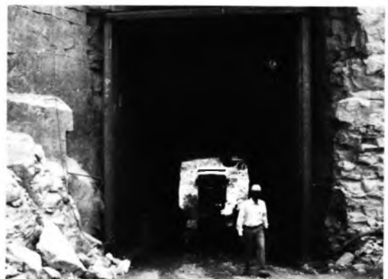
Photo. 12. Mucking through draft tube
