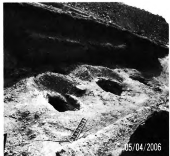
Photo. 6. Multiple shafts for delivery main
