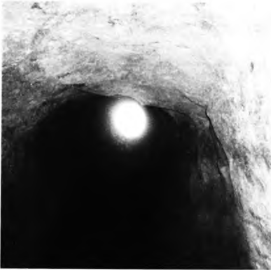
Photo. 7. Delivery main shaft
